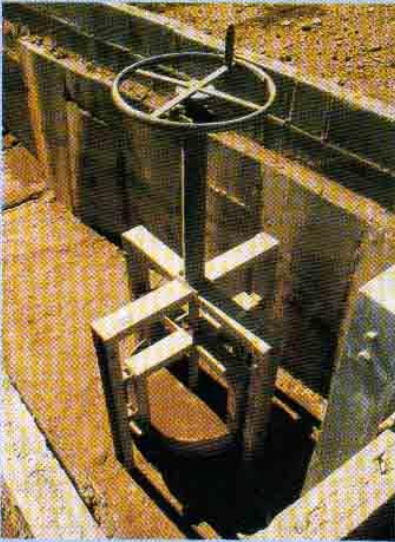
Button Gate manufactured for specific requirements. This valve seals underground pipe water flowing into farm open flume.
